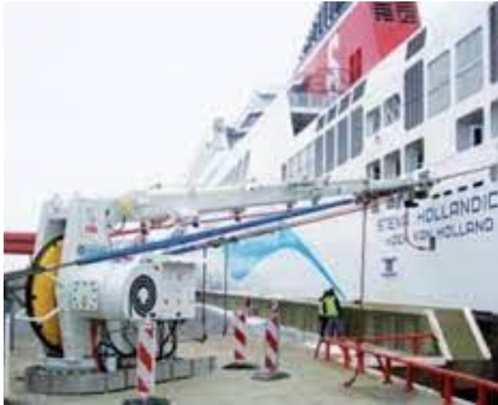
Ship plugged into shore power
